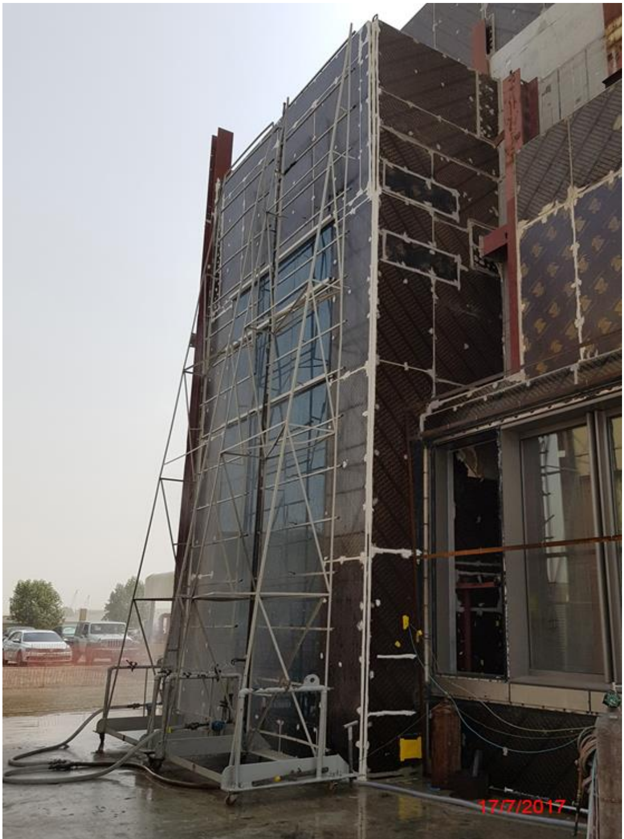
Static Water Penetration Test
