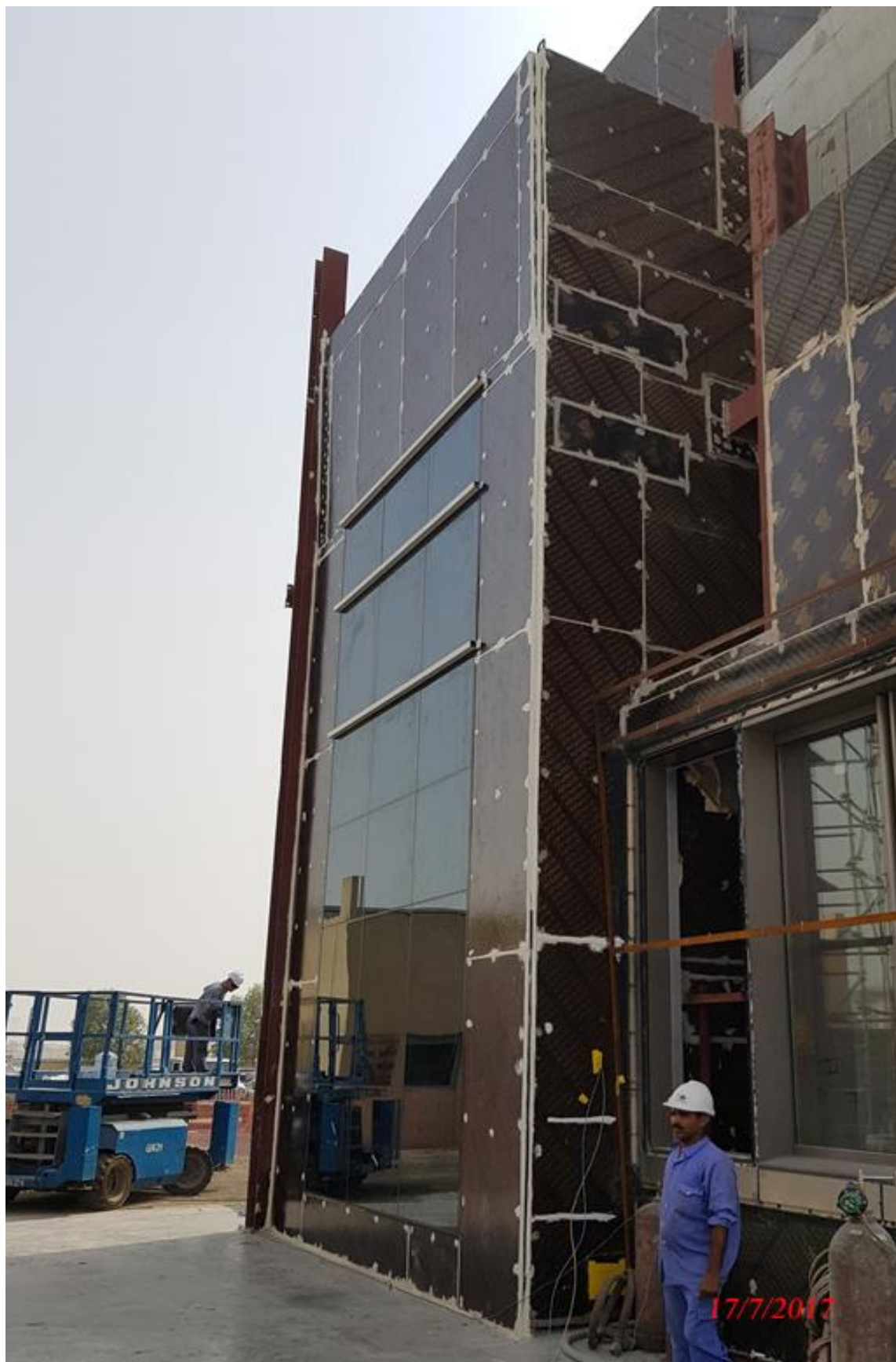
Air Infiltration – Determination of Total Air Leakage
